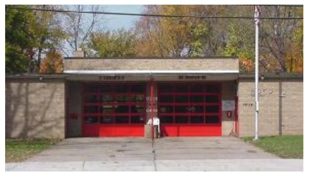
Existing Fire Station #2 on Lorain Road no longer meets the needs of the community.
