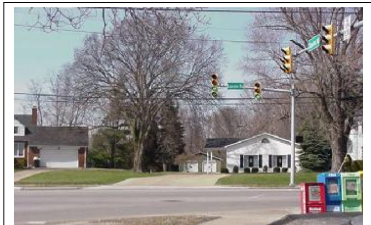
Stearns Road currently ends at Lorain Road. The project will extend the roadway north to connect to Crocker Road in Westlake.
